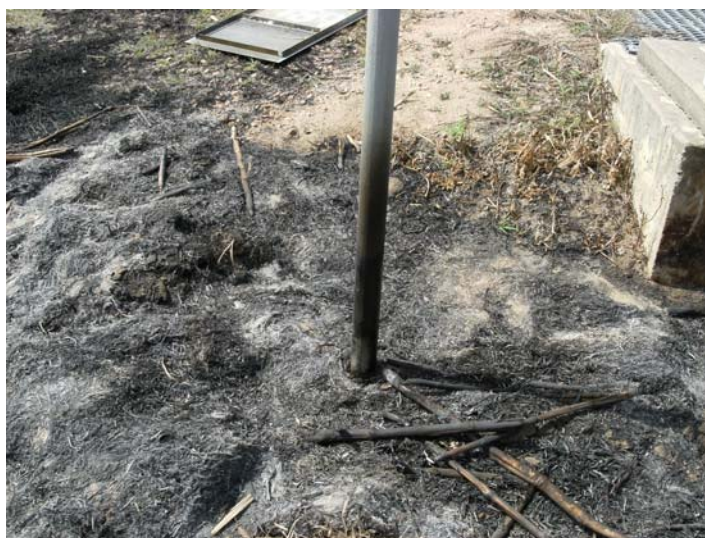
Figure 8.2: A burnt meter pole
