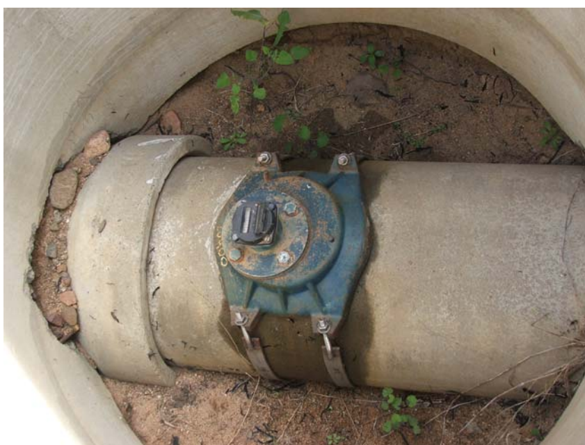
Figure 6.2: A saddle type Propeller Actuated flow meter
