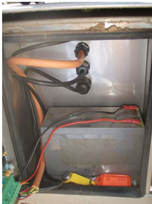
Figure 8.3: Data logger inside a display unit
