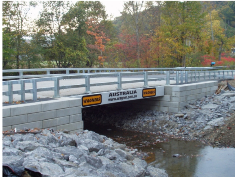
Figure 5 - Wagners Composite Bridge Deck
