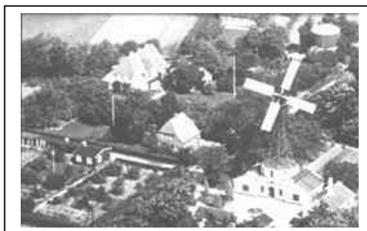
Figure 2.4 La Cour Lykkegard Turbine positioned on building.
