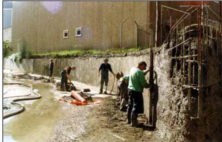
Figure 1.16: Drainage channel repair with shotcrete fibre reinforced located in Bankstown, Australia. (Source: Novocon, 2000)
