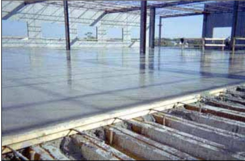
Figure 1.12: Three-storey structure in Brandon, Florida using steel Fibre reinforced slabs. (Source: Novocon, 2000)
