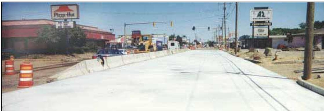
Figure 1.18: Bituminous concrete road with Fibremesh located in Springfield, Massachusetts. (Source: Novocon, 2000)
