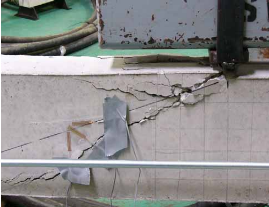
Figure 5.9: Failure Crack Pattern of Beam B2
