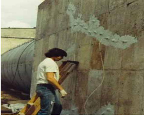
Figure1.9: Application of epoxy in tank (Source: Epoxy, 2001)
