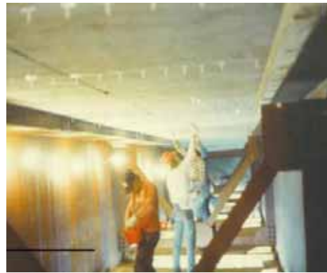
Figure1.8: Application of epoxy in slab (Source: Epoxy, 2001)
