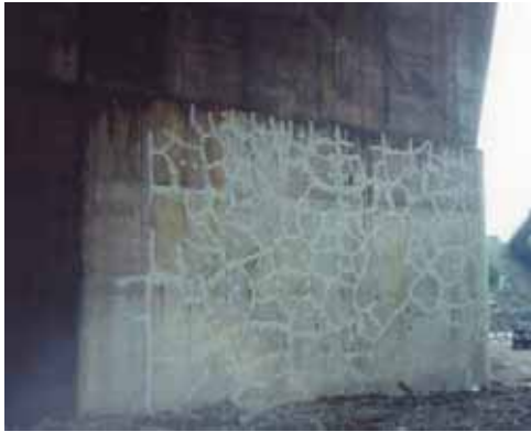
Figure1.7: Application of epoxy in wall (Source: Epoxy,2001)
