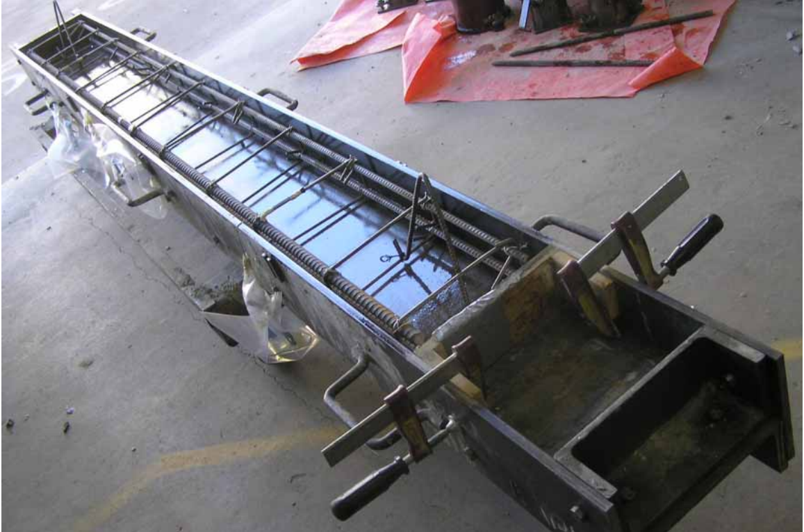
Figure 4.5: Placement of reinforcement cage in the formwork.
