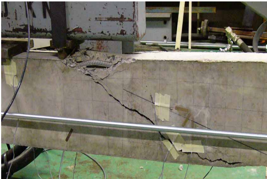
Figure 5.10: Failure Crack Pattern of Beam B3
