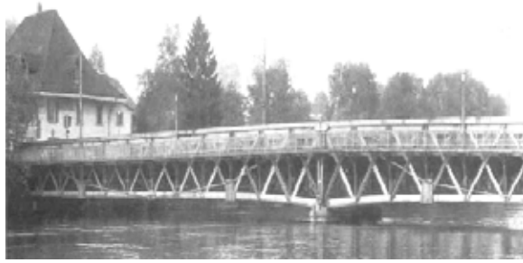
Fig 2.6: Bridge over River Aare at Aarwangen, Switzerland
