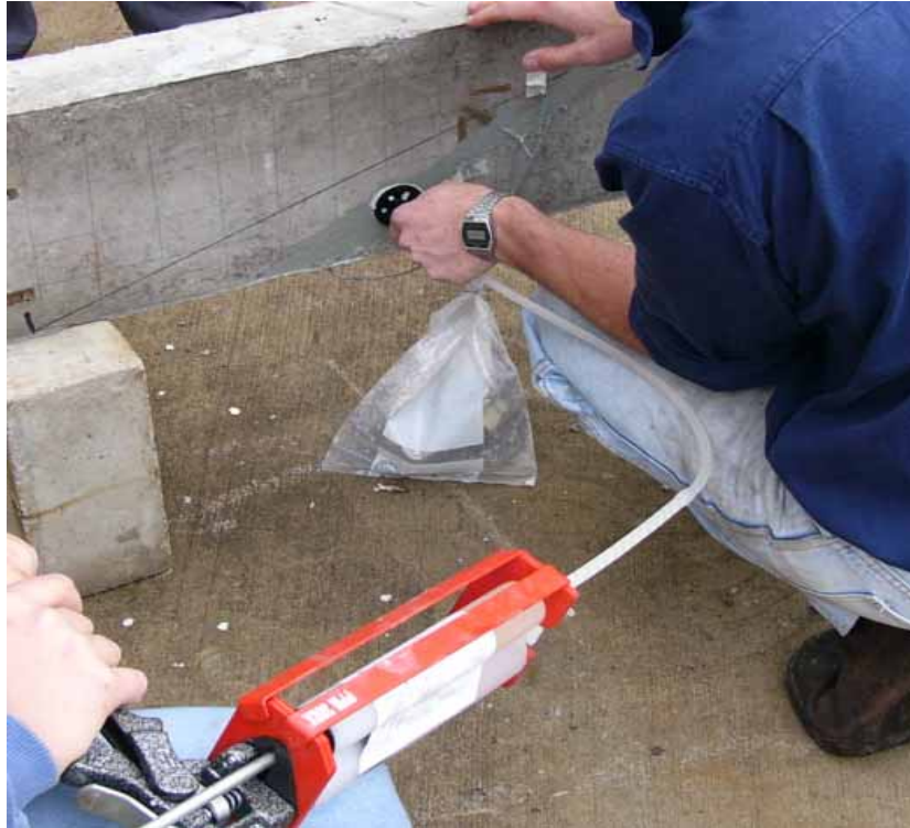
Figure 4.22: Application of epoxy in shear crack.
